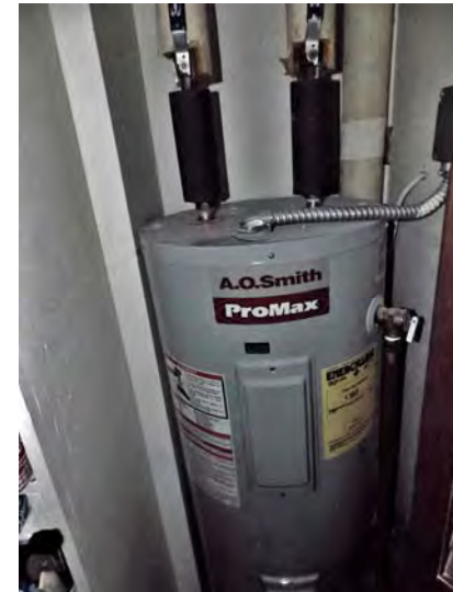
Every unit has its own electric-heated DHW tank.
