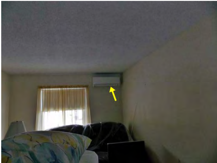
A heat pump terminal unit within one of the apartments.
