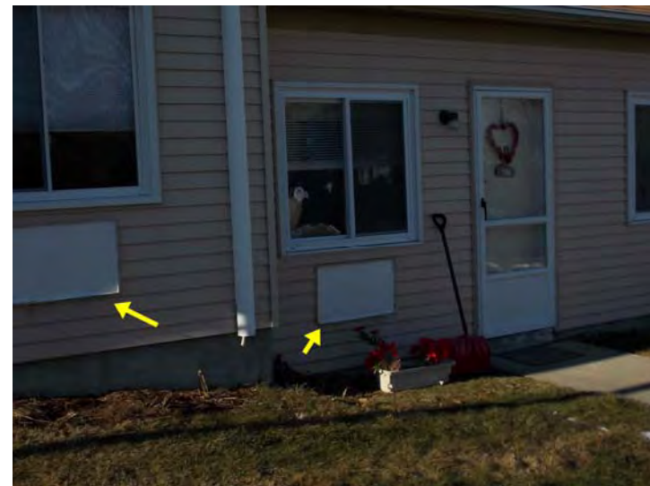
Air conditioner sleeves were being eliminated (as part of the heat pump installation project) during the site visit.
