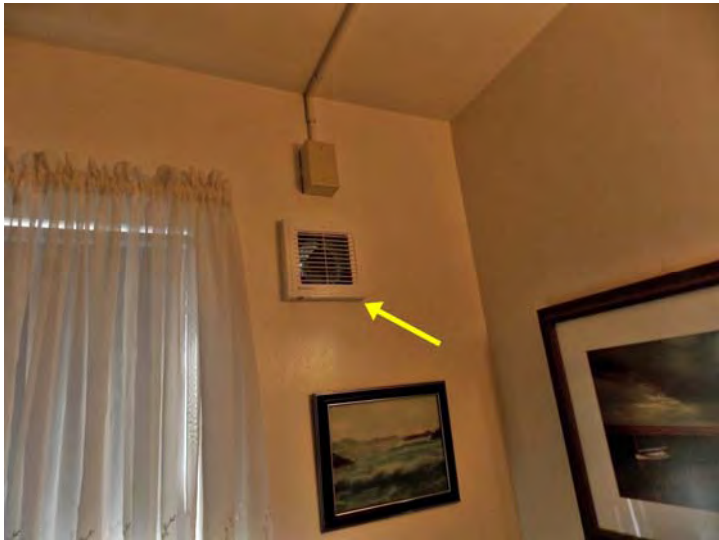
A bathroom with a wall exhaust fan.
