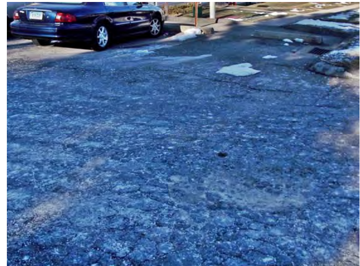
A close-up view of a damaged asphalt section.
