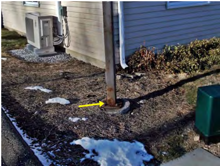
An example of a rusting light pole.
